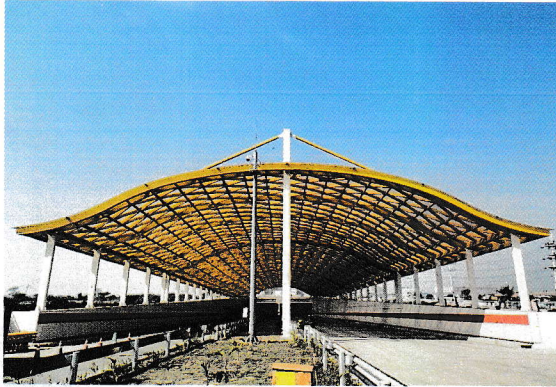
Open cut, Cut & Cover and Rain Shelter –west side:
