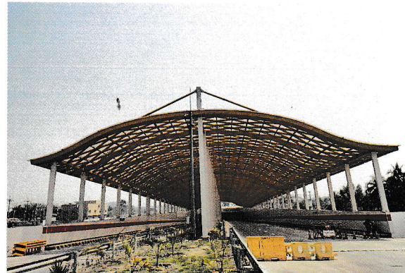
Open cut, Cut & Cover and Rain Shelter –east side:
